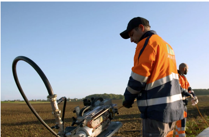
MiniXtend® cables can be placed into microducts using air-assisted equipment
