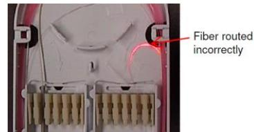
Figure 13. Bare fibers in a Splice Tray
