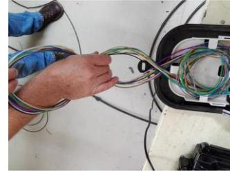
Figure 11. Storing Buffer Tubes in a Closure
