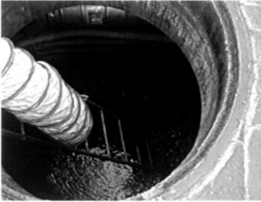
Figure 2: Conduits submerged in water inside the manhole.
