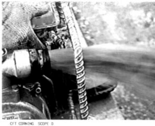
Figure 3: Water being removed from the manhole using a water pump.
