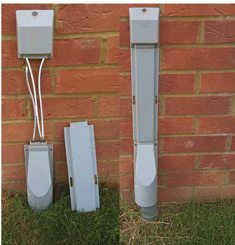
External Capping, Known as the “Elephant’s Foot”
