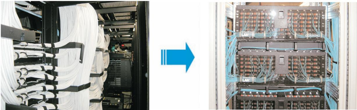
**Low density and larger copper cables (left), cause congested pathways resulting in difficult cable management and increased cooling requirements compared to compact optical fibre systems (right): both systems shown here are running at 10G**
