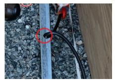
Figure 5. Examples of Installation Error Leading to Undesirable Tight Fiber Bending. Improved Resilience of G.657.A2 Compliant Fiber to Installation Errors Provides Superior Protection for the Network
