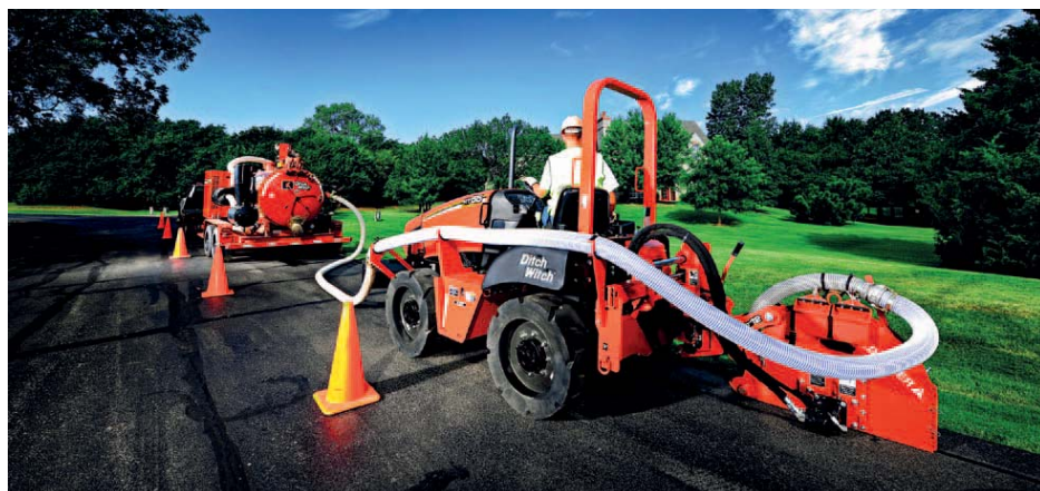
Micro-trenching is particularly suited to roadways and sidewalks where utilities are already present beneath the road surface. It requires only a shallow trench, typically about 15cm deep
