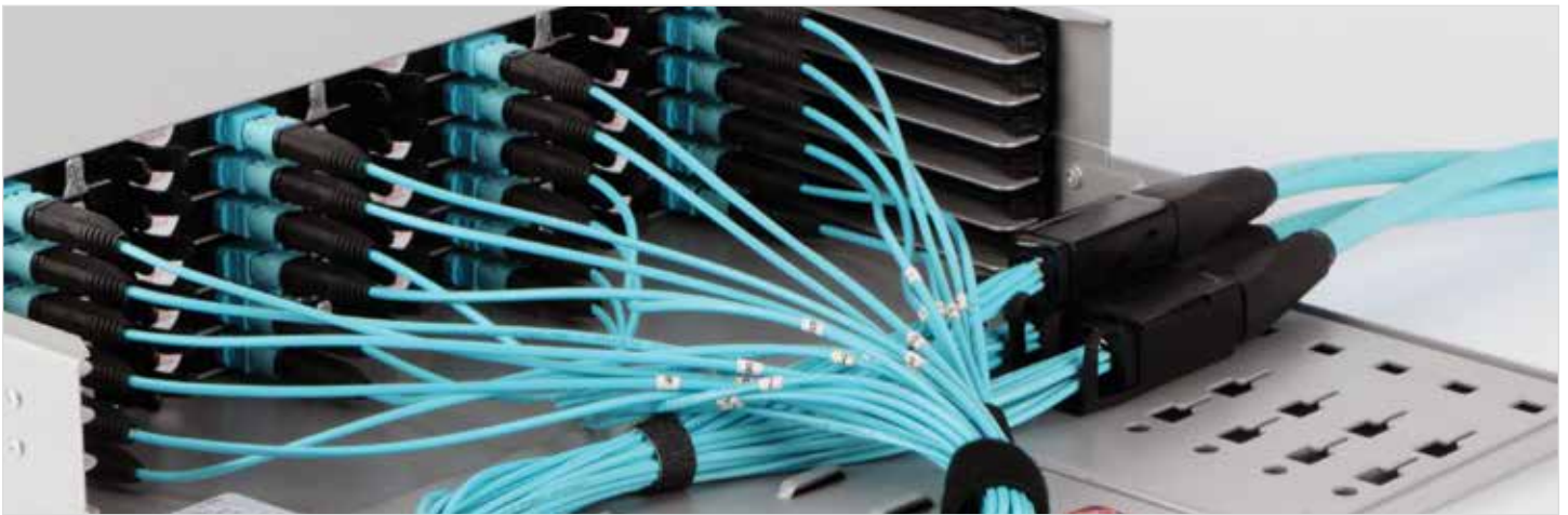
EDGE-02U Rack-Mount Rear Side | Photo LAN7314
