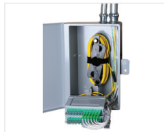
Riser Distribution Terminal Housing
