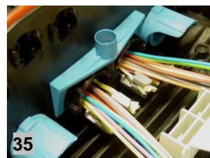
Push the tubes, micro modules or bare fibres through the double entry space (pic 34).
