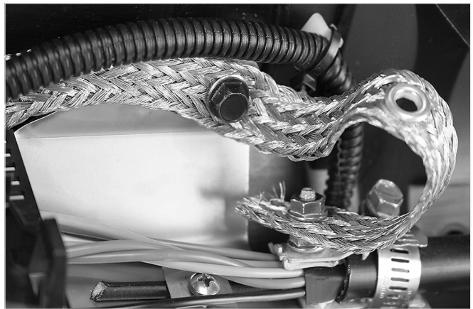
Shield Bond Connector 4460-D Installation
