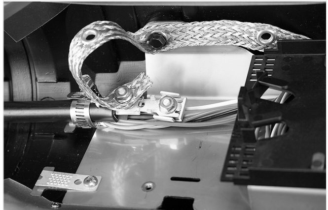
Shield Bond Connector 4460-D/FO Installation
