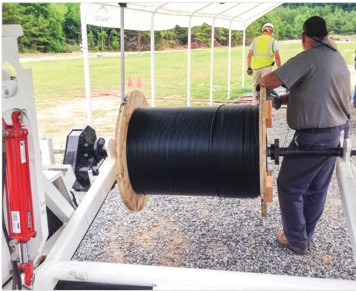
Payoff of a 144-Fiber MiniXtend® Cable
