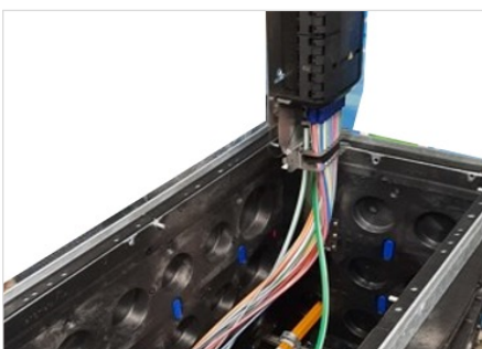
BPEO ECAM with Gasstop Installed on Mobile Bracket (MOBRA) in Manhole
