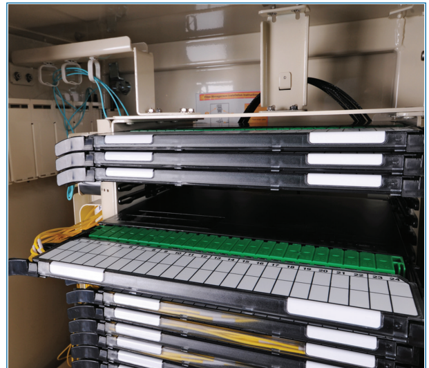
OptiTest HD Cabinet, 896-Fiber, Pad Mount (Centrix Cassette) | Photo CRR2429
