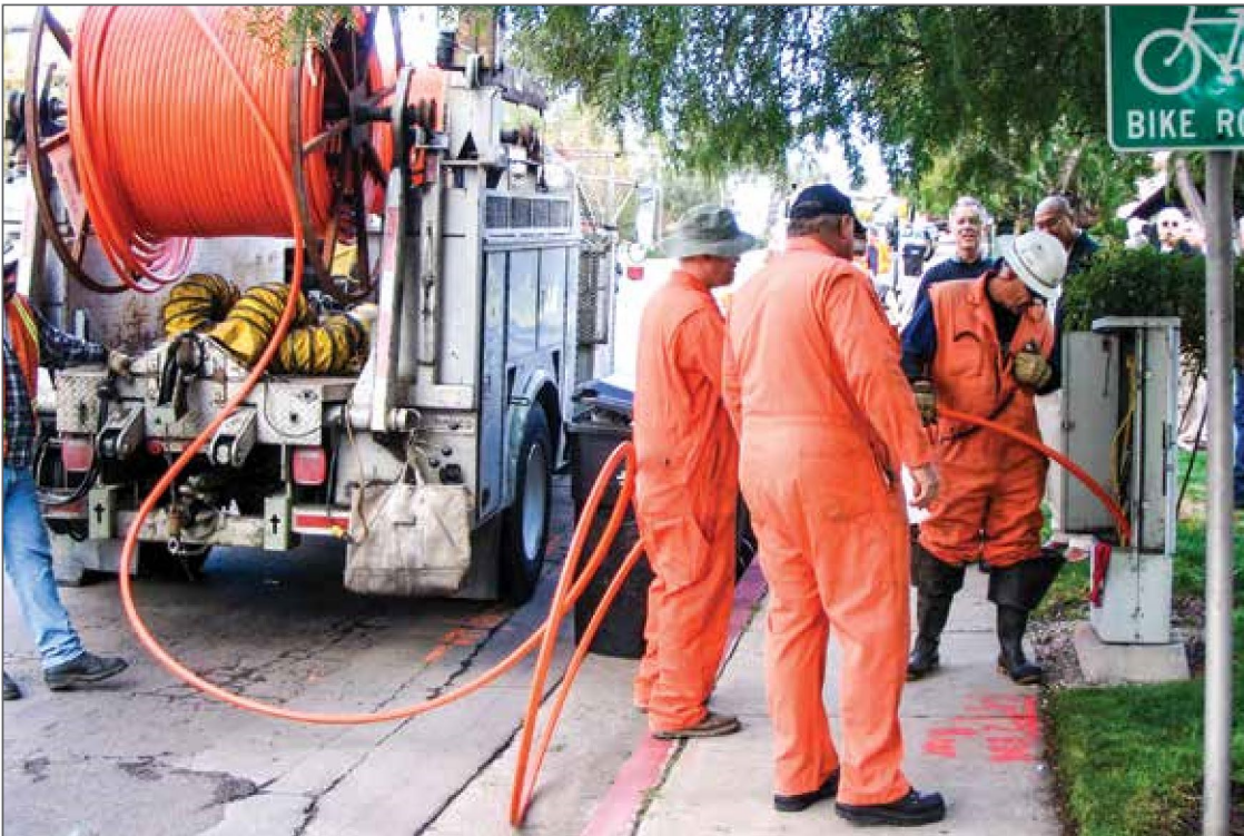
Figure 1. Microduct installation
