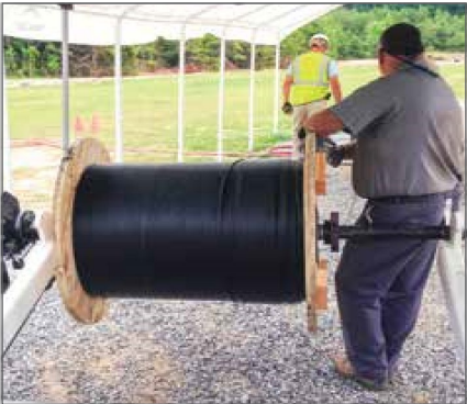
Figure 7. Payout of a 144-Fiber MiniXtend Cable
