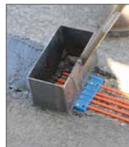
Figure 33. Microtrenching Method
