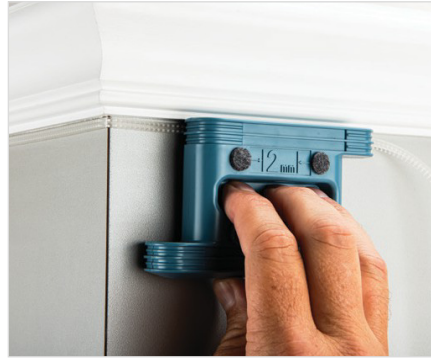
Installation of Hallway Fiber Pathway with Clear Track Hallway Universal Installation Tool
