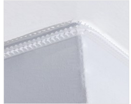
Clear Track Hallway Fiber Pathway Installed Around Exterior Corner
