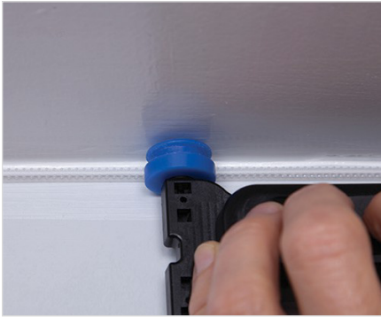
Installation of Clear Track Hallway Fiber Pathway with Hallway Installation Tool
