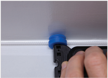
Installation of Clear Track 12-Fiber Micro-Module Into Clear Track Hallway Fiber Pathway
