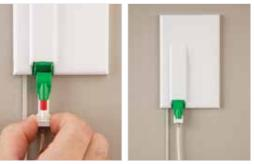
First, we cleared the room. Now, we're clearing the hallway. Corning<sup>®</sup> Clear Track Hallway Fiber Pathway The Corning<sup>®</sup> Clear Track Hallway Fiber Pathway is the virtually invisible way to deliver ultra-high-speed Gigabit broadband to multidwelling units (MDUs). It adapts micro-replication technology for the multifiber needs of MDU hallways to enable fast and easy installation with minimal disruption for
