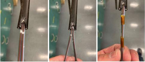
Next, slide a piece of 1" pre-shrunk ID heat shrink tubing over the cable jacket. Then slide the split mesh tubing into place and carefully heat the furcation. This creates a very robust and safe solution for keeping the ribbons protected while being routed and spliced inside a closure.
