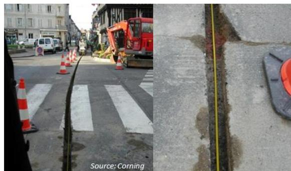
**Figure 4. Example of microtrenching deployments in urban areas**
