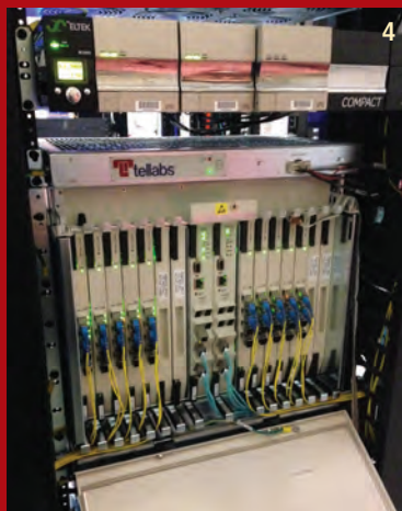
1) Zone location in back of house. 2) Optical fibers hardly take up any space in an old-design cable tray. 3) Corning ONE DAS headend equipment. 4) Optical line terminal (ONT) in Kyle Field MDF. 5) Kyle Field command center. (Photo 2: Corning. All other photos this page: IBM/Texas A&M)
