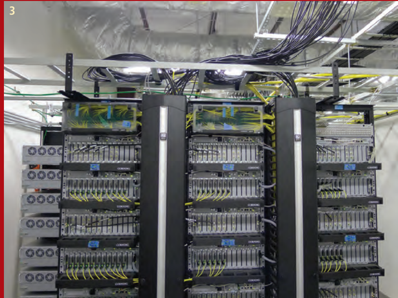
1) Zone location in back of house. 2) Optical fibers hardly take up any space in an old-design cable tray. 3) Corning ONE DAS headend equipment. 4) Optical line terminal (ONT) in Kyle Field MDF. 5) Kyle Field command center. (Photo 2: Corning. All other photos this page: IBM/Texas A&M)
