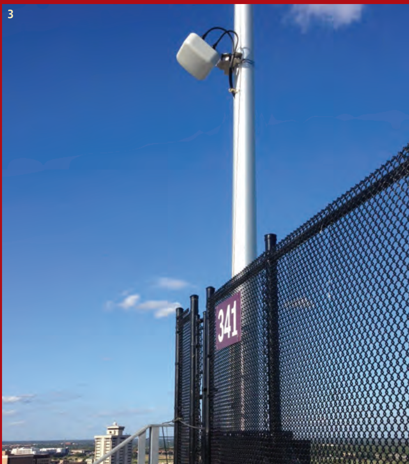
1) Kyle Field scoreboard. 2) Zone location and antenna under overhang. 3) Upper bowl zone box (remote gear) and directional antenna. (All photos this page: IBM/Texas A&M)
