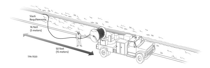
Verify that sufficient slack for splicing is available before securing the cable in the trench. Position the cable at the starting location, aligning the appropriate PAM marker with that location. The cable may need to be temporarily secured to prevent transition as the reel is driven off.
